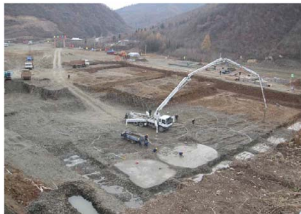
Pouring concrete foundations for CIL tanks
