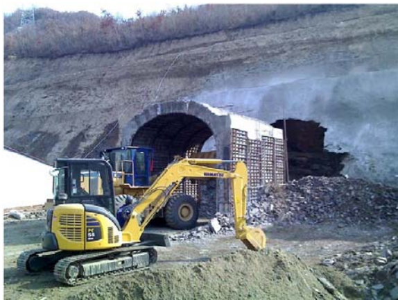
First firing at decline portal
