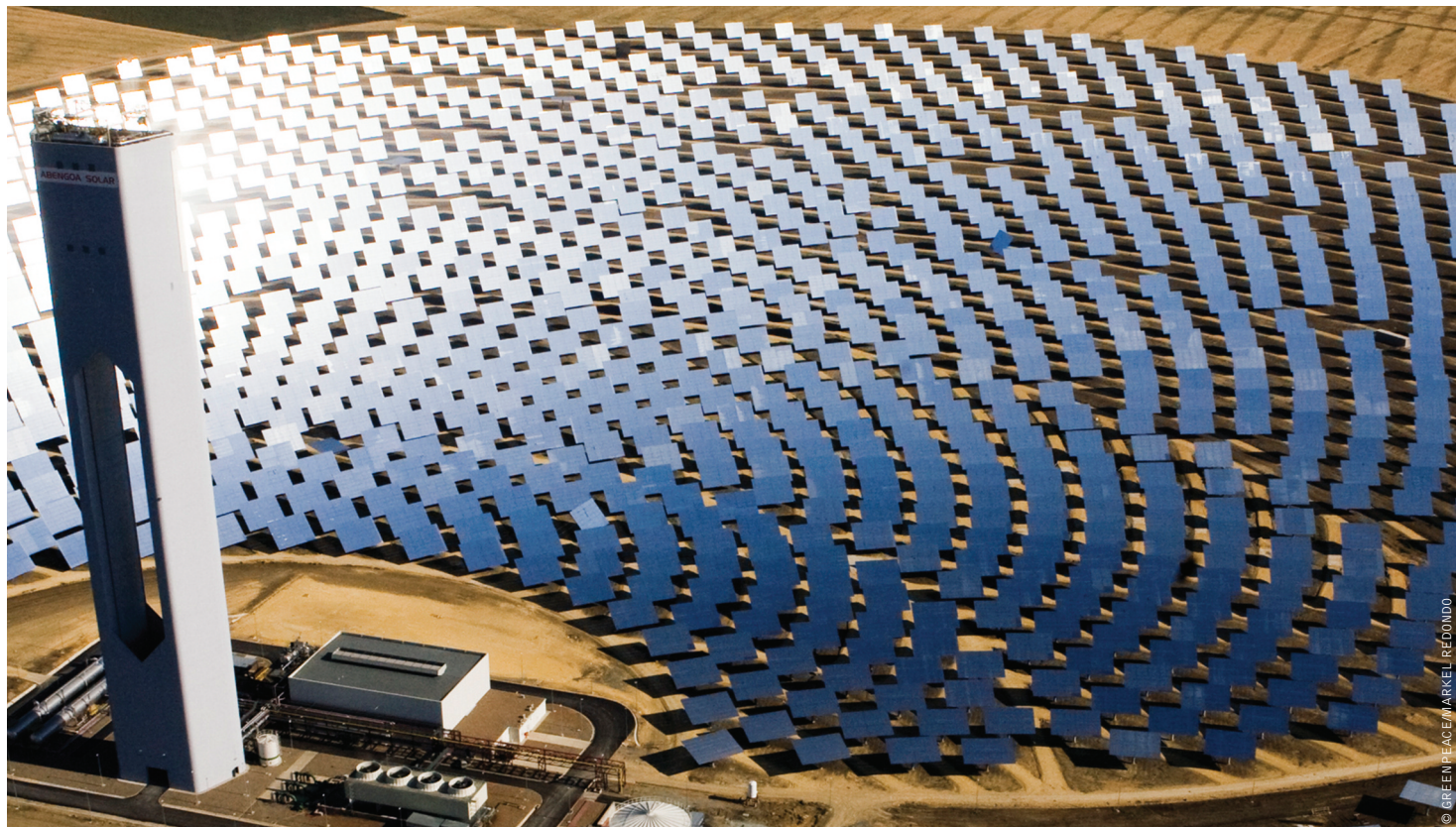
image THE PS10 CONCENTRATING SOLAR THERMAL POWER PLANT IN SEVILLA, SPAIN. THE 11 MEGAWATT SOLAR POWER TOWER PRODUCES ELECTRICITY WITH 624 LARGE MOVABLE MIRRORS CALLED HELIOSTATS. THE SOLAR RADIATION, MIRROR DESIGN PLANT IS CAPABLE OF PRODUCING 23 GWH OF ELECTRICITY WHICH IS ENOUGH TO SUPPLY POWER TO A POPULATION OF 10,000.
