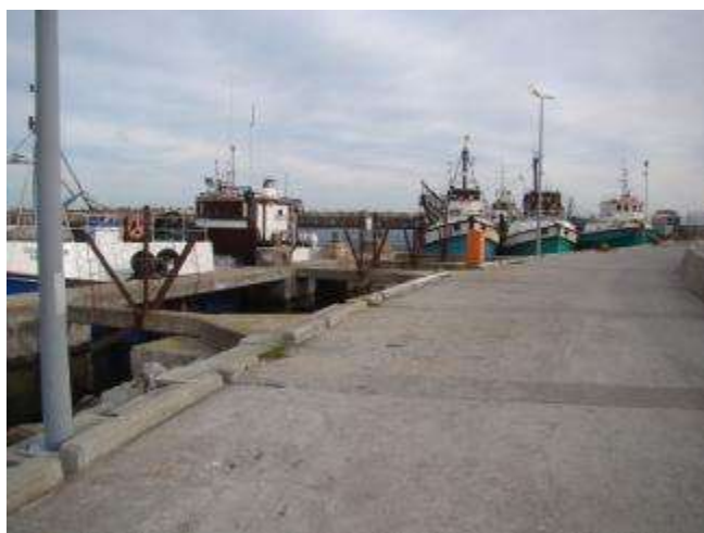
Figure 82: Berthing quays north harbour
