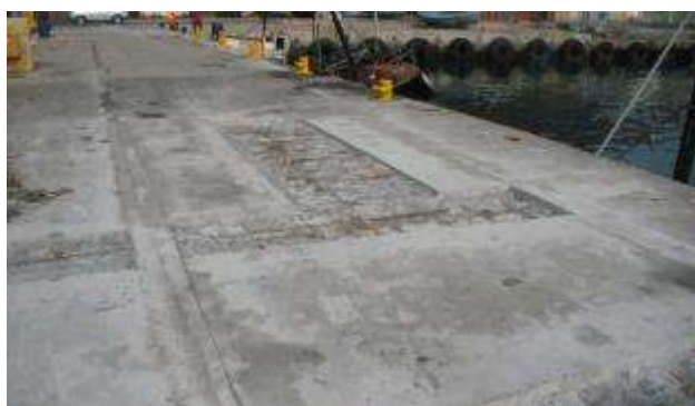
Figure 45: Repair quay surface
