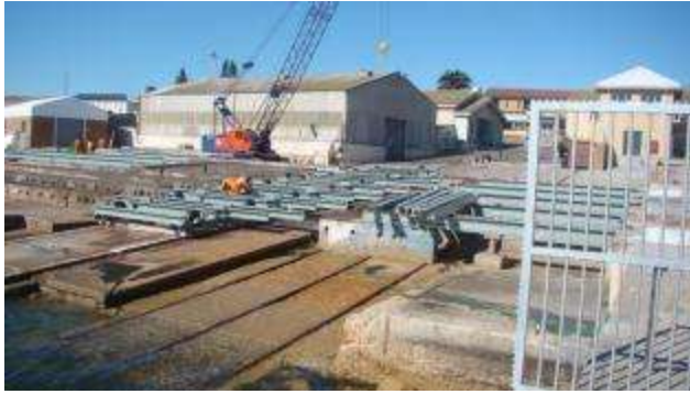
Figure 9: Cradle on slipway being refurbished
