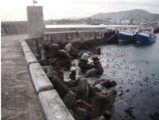
Figure 86: Inside of outer breakwater
