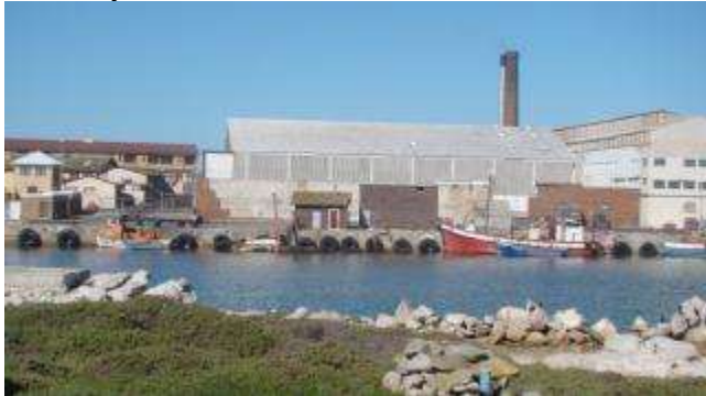
Figure 6: View onto jetty
