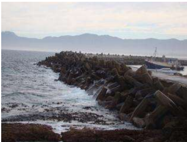
Figure 85: Outer breakwater external
