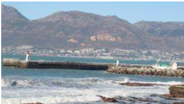
Figure 52: Breakwaters with a fishing vessel berthed on the outer breakwater
