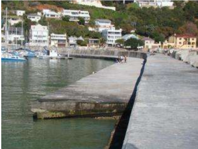
Figure 59: South breakwater internal
