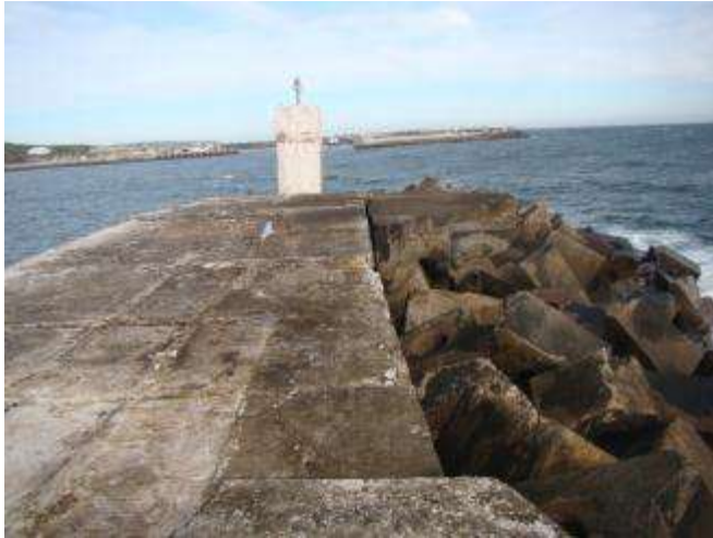
Figure 88: South harbour outer breakwater
