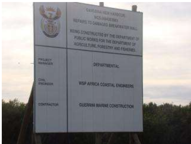
Figure 87: Contractors notice, north harbour
