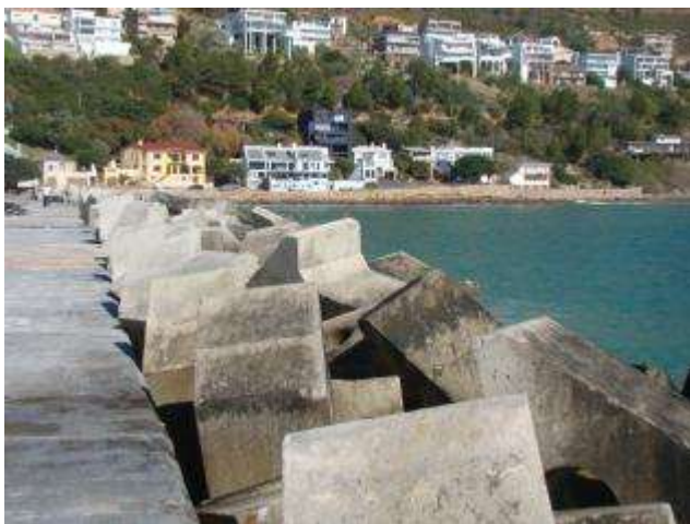
Figure 60: South Breakwater external
