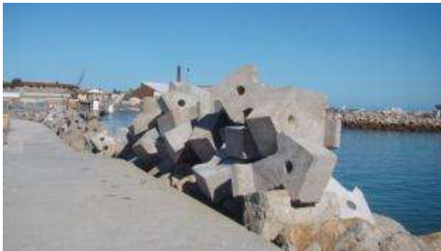
Figure 10: New mini dolloss being placed
