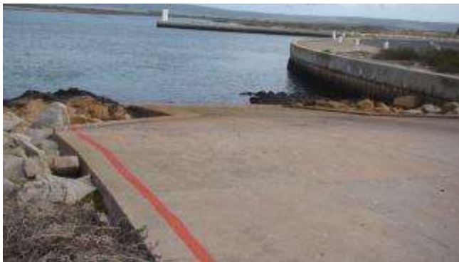
Figure 36: Small craft slipway
