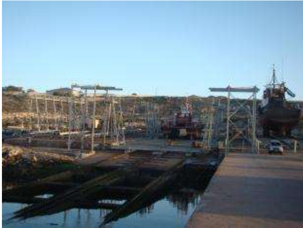
Figure 29: Slipways and cradles
