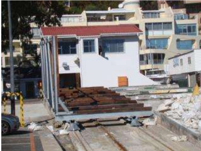
Figure 63: Cradle and slip under maintenance
