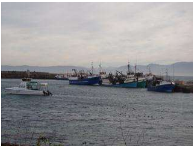
Figure 80: North (new) harbour with quays and anchorages
