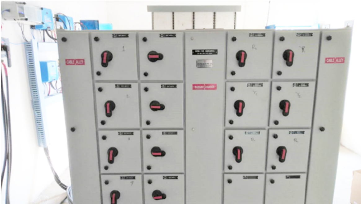
Figure 32 Mlinda-designed DCDB: Catered to allow for three increases of capacity from 23.6 kWp to 38.6 kWp
