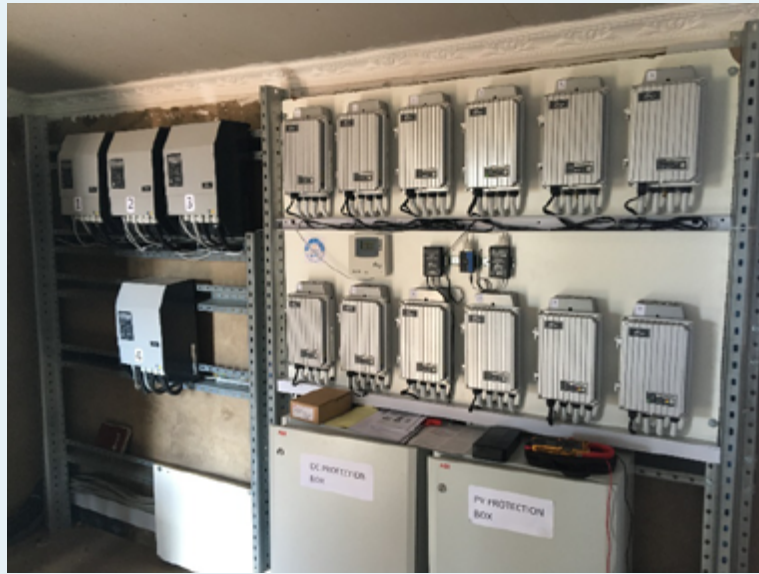
Figure 39 Inverters and MPPT solar controllers
