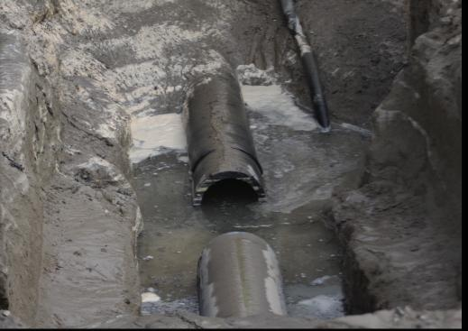
When this generator needed to make an urgent repair to a 18" | 450 mm HDPE water supply line, they needed a solution that could guarantee a fast return to service, regardless of site conditions or weather.
