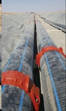
When considering a pipe joining method for their 2.5 mile | 4 kilometer long, 24" | 630 mm OD HDPE tailings pipeline at Husab Uranium Mine, the Husab Joint Venture sought a solution that would allow for ease of future maintenance and a fast initial installation.
