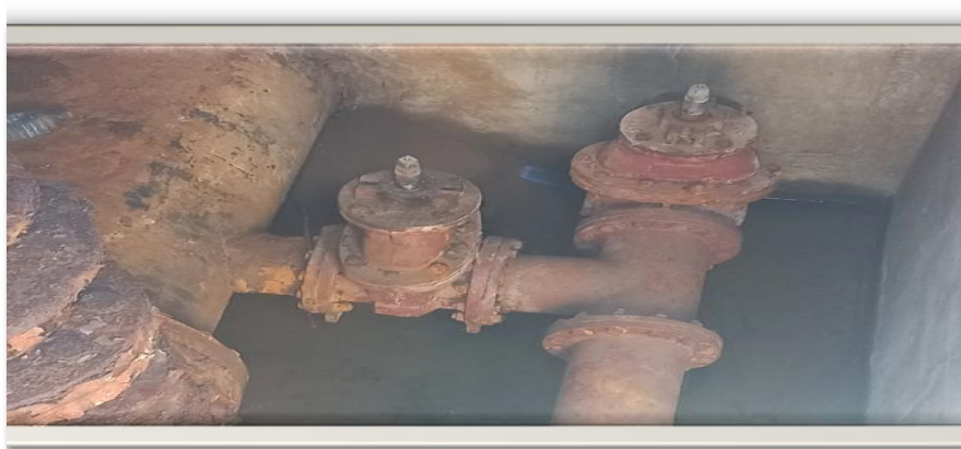
Photo A: depicts a visibly rusty and dilapidated water isolation valve inside the concrete chamber next to Amanzimtoti pumping station
