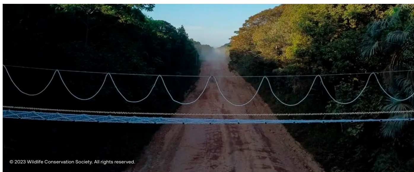
Figure 6.3 Construction of a canopy bridge for primates
