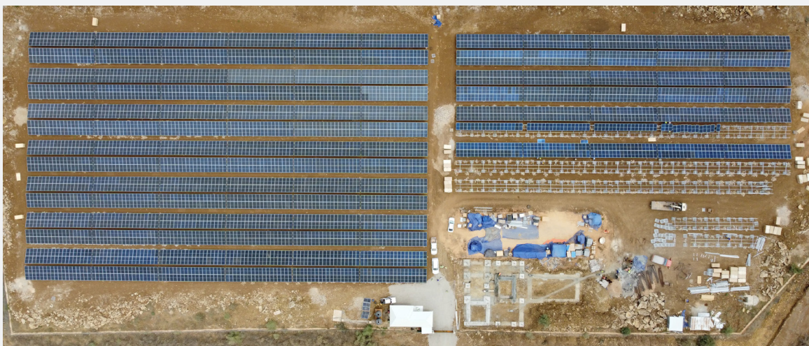
Figure 5 Construction phase of the solar power project in Baidoa
